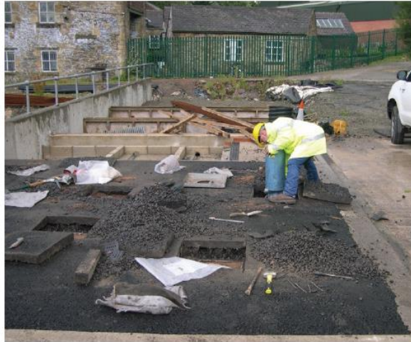
Figure 3 - In situ density tests post-trafficking.
