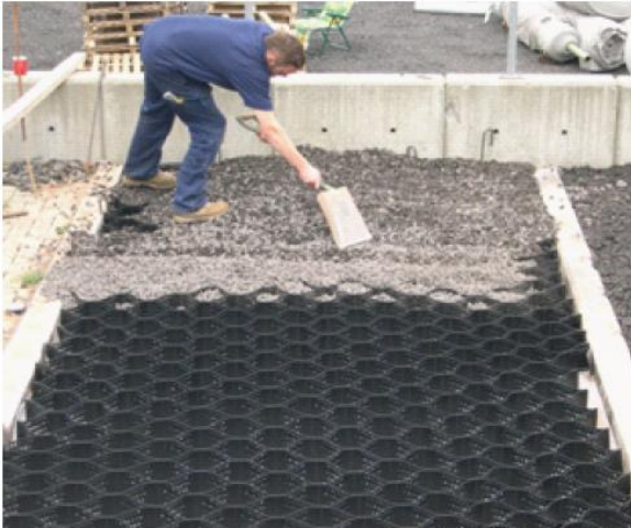
Figure 2 - Cellweb TRP® in construction.
