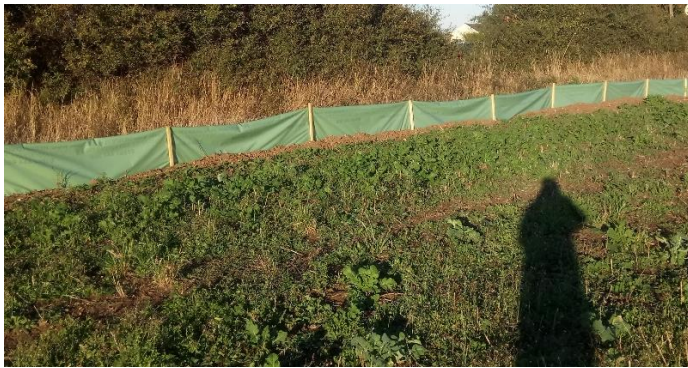
Figure 3: example image of non-permanent 'drift' herptile fencing
