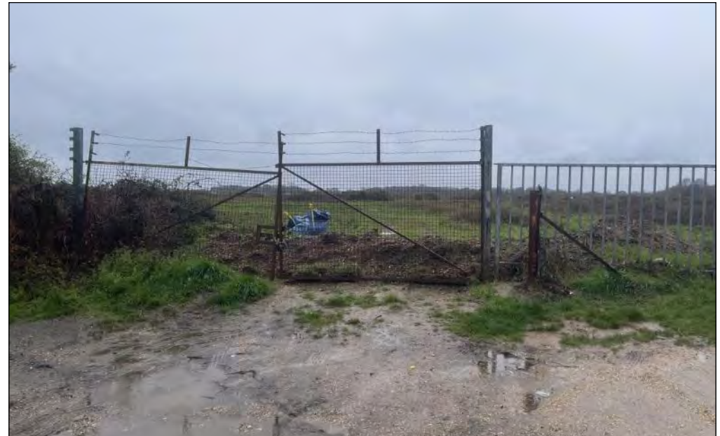
40. Road Access Gates
